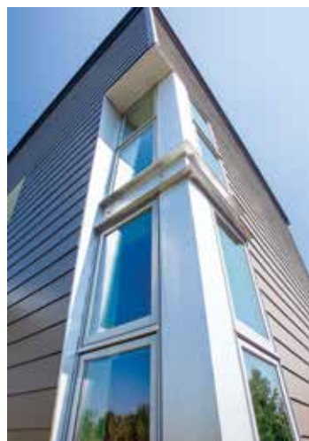
This gradually recessed window well makes the most of the sun's light and radiant heat.
